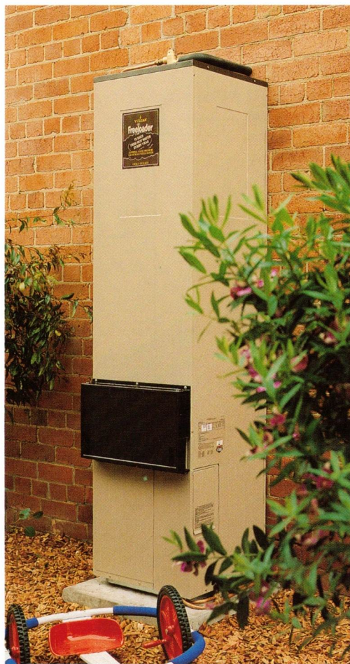
Unit installed on concrete slab.
