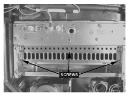
f. Remove two (2) burner retaining screws, then remove combustion chamber front panel (9
