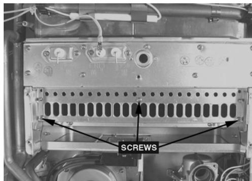
f. Remove two (2) burner retaining screws, then remove combustion chamber front panel (9 screws).
